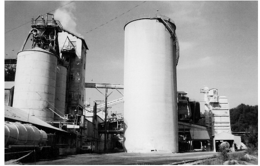
The 120-foot concrete storage bunker known as No. 6 in the center of this photograph was built in 1936. It has a maximum capacity of 10,000 tons but currently holds about 7,000 tons of finished lime. The area where lime is weighed and loaded into trucks for bulk
