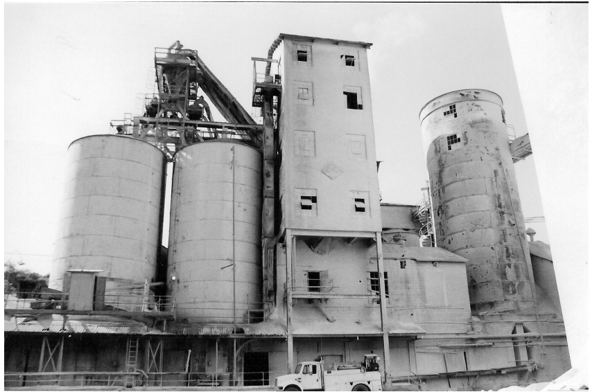
This group of buildings includes the 100-foot hydrating plant in the rectangular building in the center, the "12-foot classifier" where the pebble lime is sorted by size in the round building on the right, and two 75-foot lime storage bunkers on the left. All of these structures were built between 1922 and 1931, when the American Lime and Stone Company was under the management of Warner Company.
