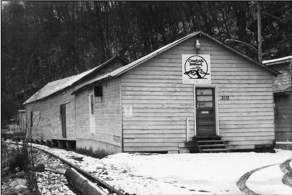
VIEW OF THE EAST END OF THE SUCKER STICK FACTORY, LOOKING WEST.
