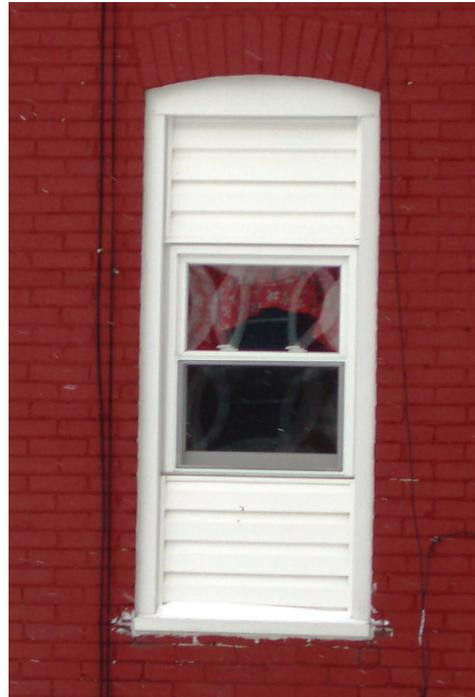
*This window was replaced with no regard for matching the size, shape, or materials. It is likely that the muntin pattern was much different on the original window.*
