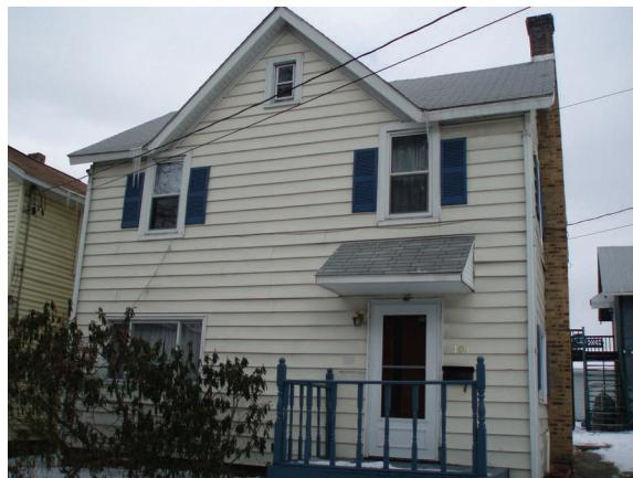
*The shutters on the second story of this home are not proportioned correctly. They seem to float in the middle of the window.*
