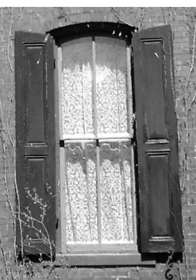
*Note how these shutters are scaled to match the window. They are curved at the top to match the shape of the window.*
