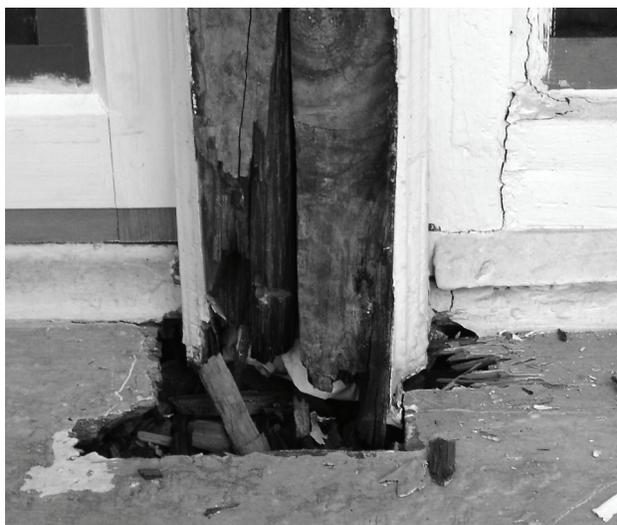
*The decay in this window could have been discovered sooner with a routine window inspection.*
