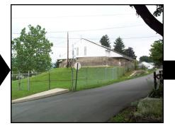
From this reservoir, water is then gravity fed to a portion of the town's customers. Like the Big Spring, the reservoir is covered to protect the water quality. Water is also pumped to the standpipe on Hughes Street.
