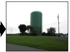
A second holding facility is located on the south side of the borough on Hughes Street behind the high school football field. Water from the large, blue tank is gravity fed to the remaining portion of the borough. Some lines do extend outside the borough. At various points in the system, small pump stations exist to add pressure for the water system.
