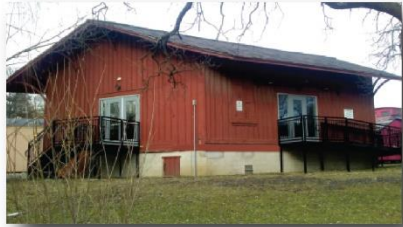
View from park showing door locations
