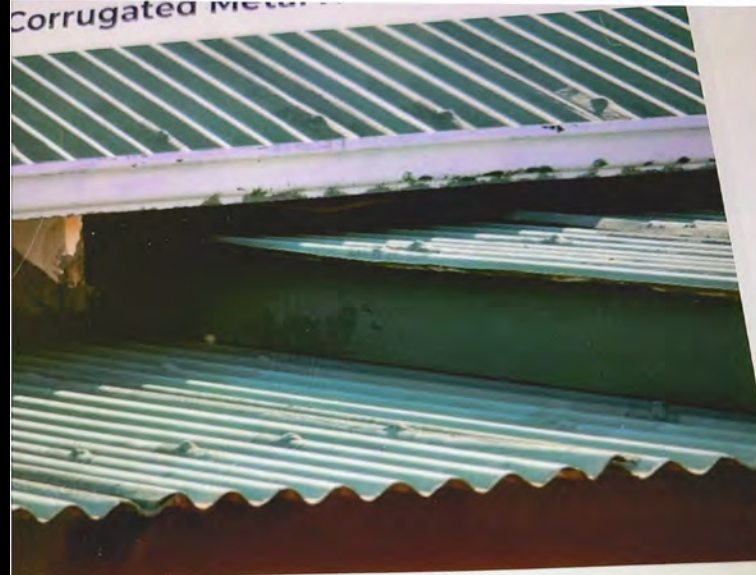
Sections of corrugated metal roofing were not galvanized nor
