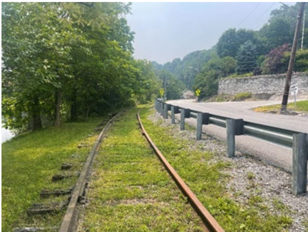
Figure 9 (top): South Potter Street with newly installed signs signal to drivers that pedestrians are present. Figure 10 (bottom): Former railbed along South Potter is an opportunity and could be converted as a multi-use path that connects Talleyrand and Masullo parks.
