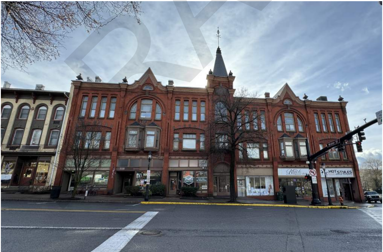
Bush Arcade (224 West High Street), constructed in 1887.
