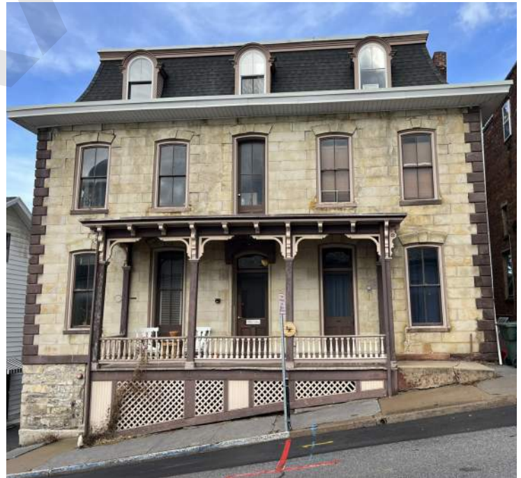
119 East High Street; construction date unknown
