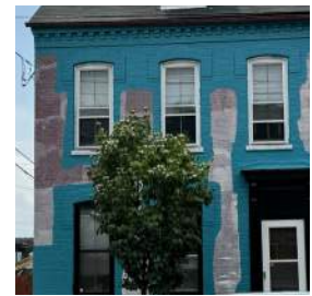
Example of inappropriate use of paint on masonry substrates, as well as inappropriate color choice
