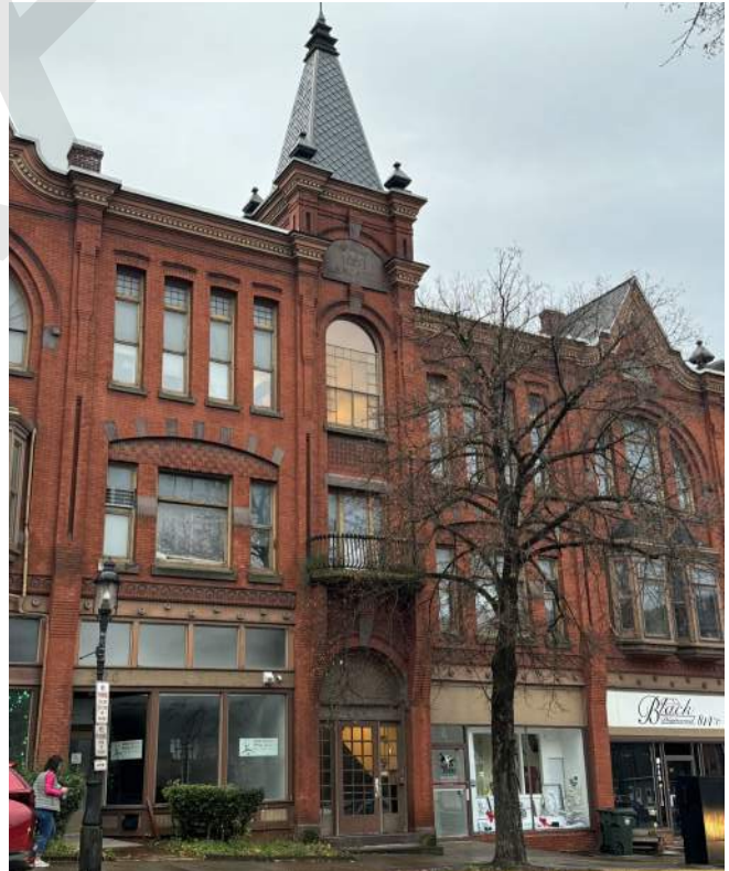
Bush Arcade (216-226 W High Street; constructed in 1887)
