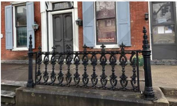
Example of an iron fence at 140 W High St.
