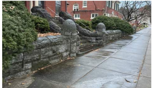
Example of a stone retaining wall at 222 N Allegheny St.
