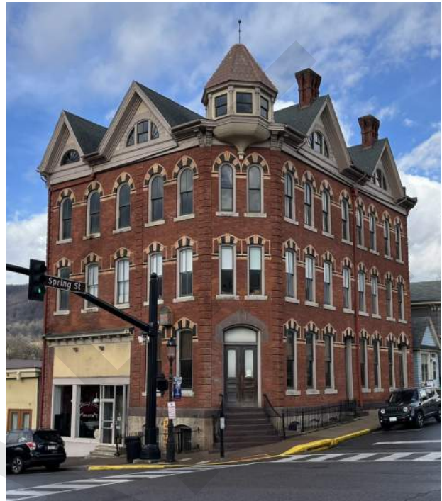
Centre County Banking Co. Building (201 West High St.; 1881).
