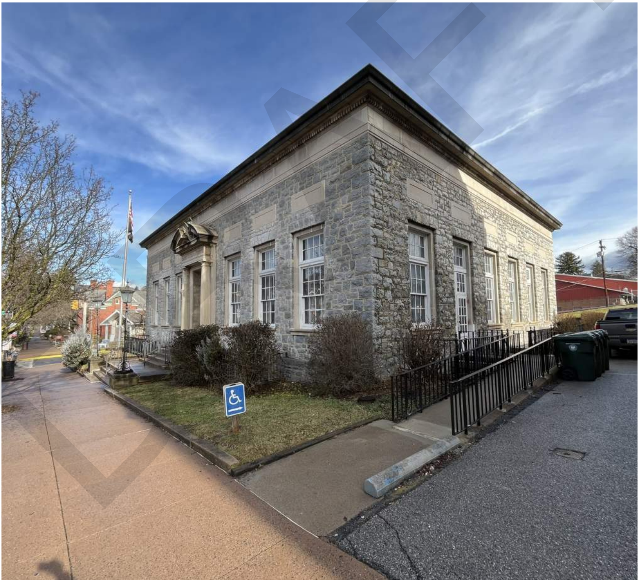
Historic Post Office (132 North Allegheny Street), constructed in 1935 with the familiar limestone walls of older Bellefonte buildings.
