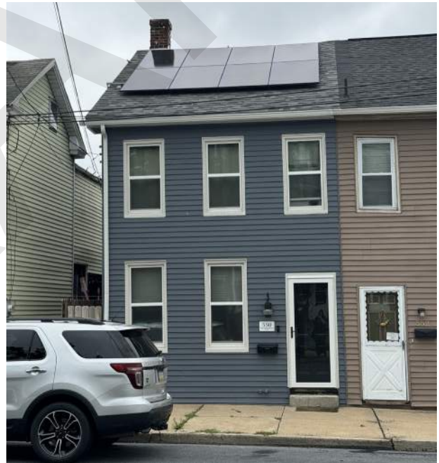
Example of inappropriate solar panel installation on roof slope easily seen from right-of-way.
