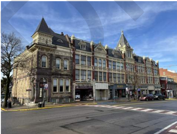
Streetscape along 101-117 N Allegheny Street
