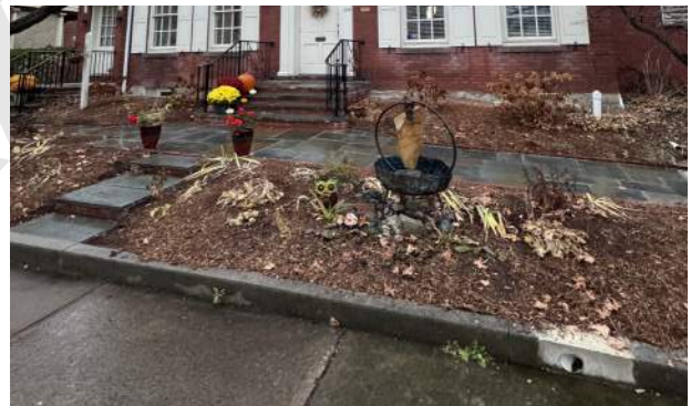
Example of a character defining walkway at 214 N Allegheny St.
