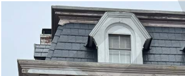
Roof replacement utilizing substitute material to replicate original historic slate material
