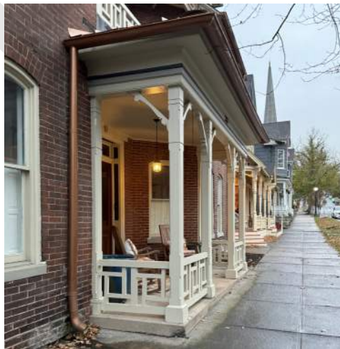
Example of an original wood porch with railing at 233 N. Allegheny Street
