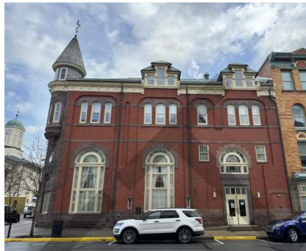
W.F. Reynolds & Co. Bank Building (108 S Allegheny St; 1887).
