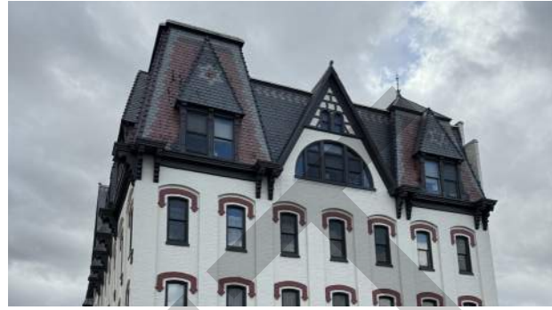
Example of an original slate roof at the Brockerhoff House Hotel
