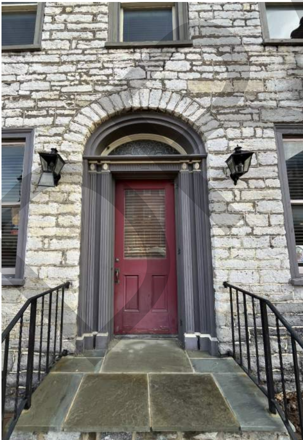
Original limestone house at 124 North Allegheny Street, dating from c. 1835 and built in the German Colonial tradition.
