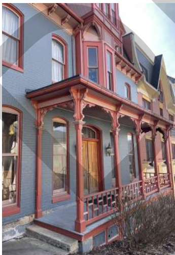
Example of an original wood porch with railing at 119 E. High Street.
