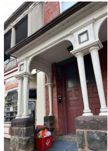
Example of an original wood porch with stone foundation walls at 132 W High St.
