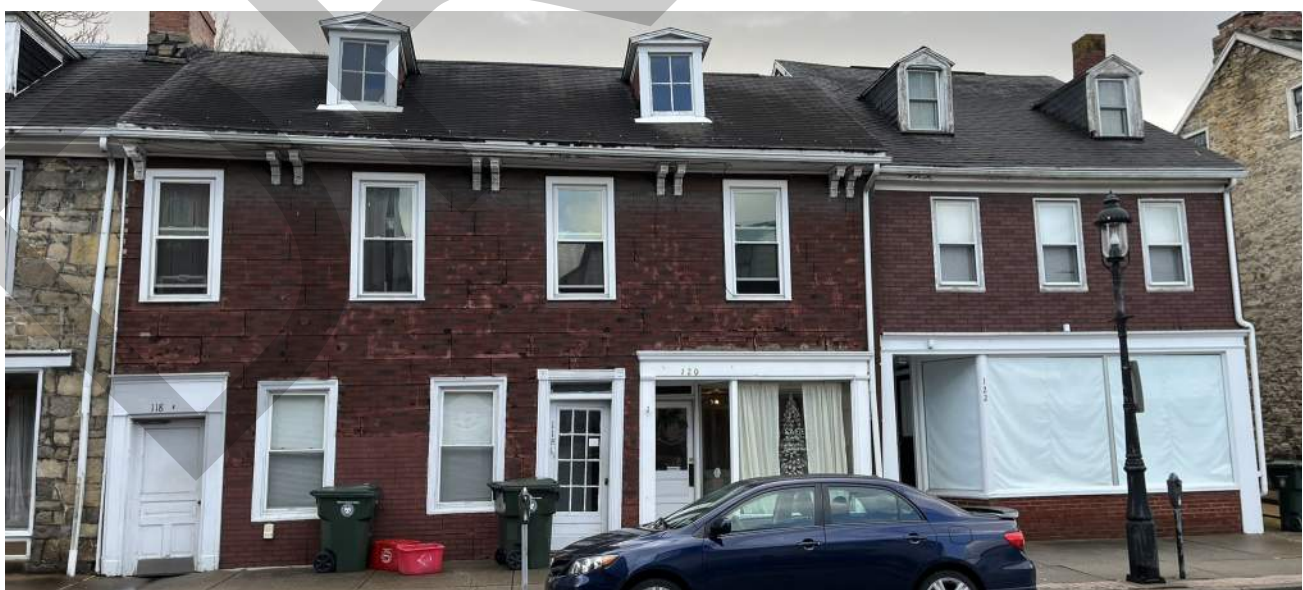
118-122 West Bishop Street; construction date unknown
