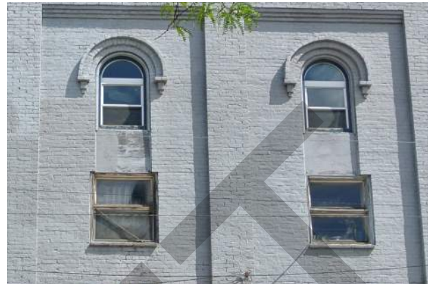
Example of replacement windows that are inappropriate and do not meet the guidelines
