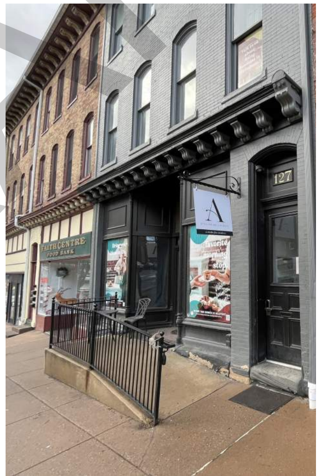
127 South Allegheny Street; construction date unknown
