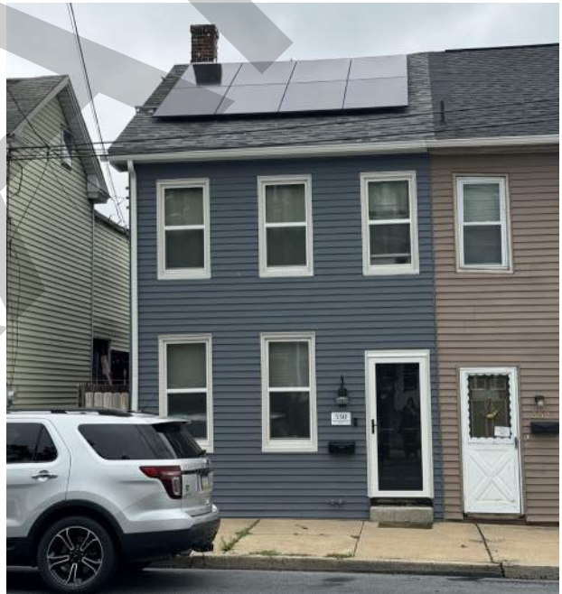
Example of inappropriate solar panel installation on roof slope easily seen from right-of-way.
