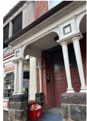
Example of an original wood porch with stone foundation walls at 132 W High St.
