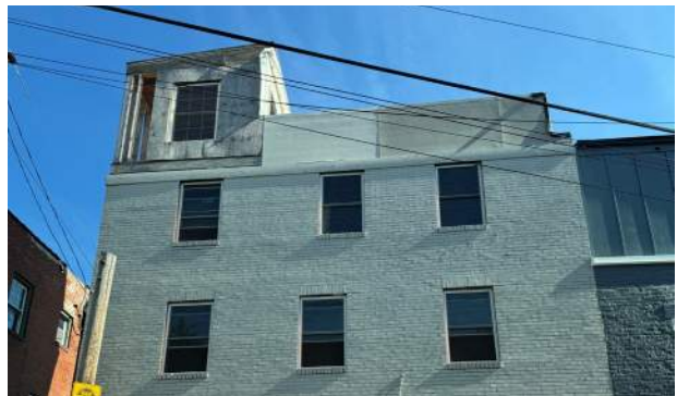
Example of an inappropriate rooftop addition.
