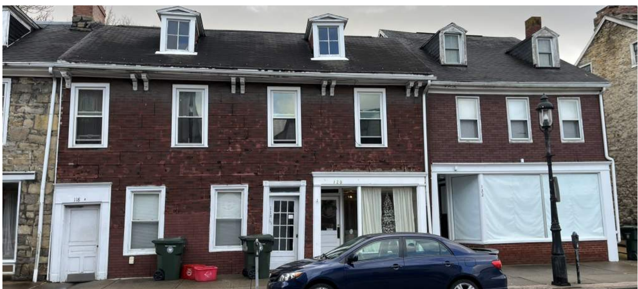
118-122 West Bishop Street; construction date unknown
