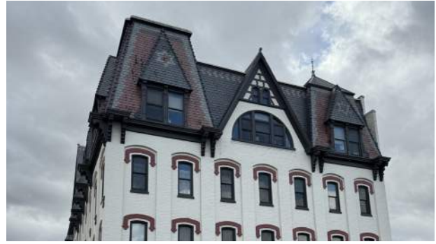
Example of an original slate roof at the Brockerhoff House Hotel
