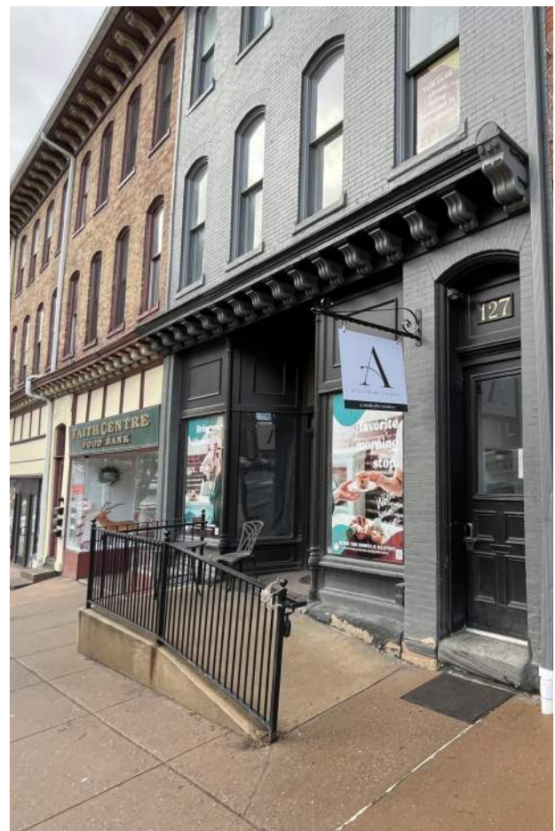
127 South Allegheny Street; construction date unknown
