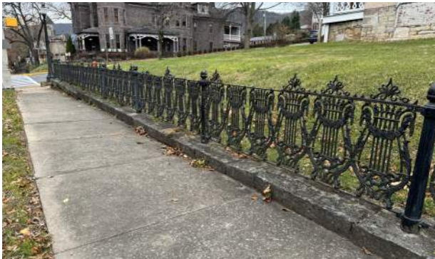
Example of an iron fence at 107 E Linn St.
