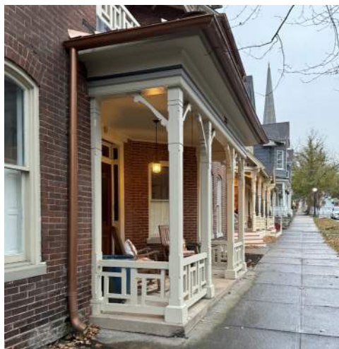
Example of an original wood porch with railing at 233 N. Allegheny Street
