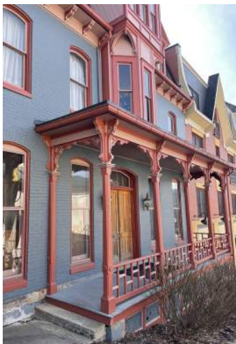
Example of an original wood porch with railing at 119 E. High Street.
