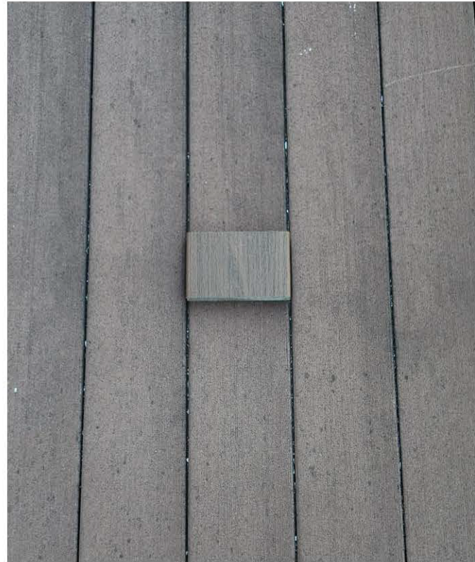
Sample of Trex “Hatteras” decking overlaid on the current composite deck.
