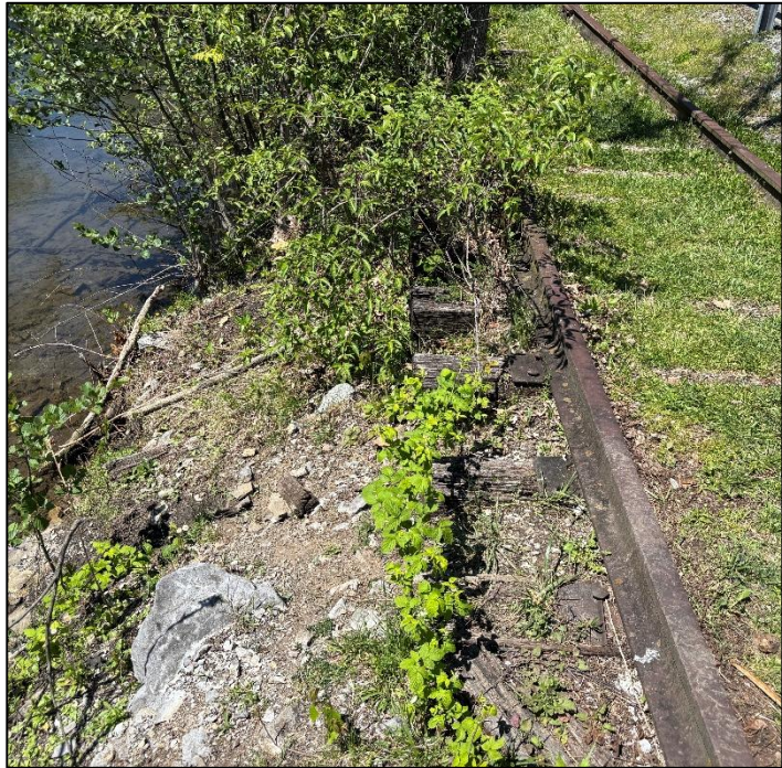
Photo 6 – Corridor encroaching on Spring Creek, Looking West
