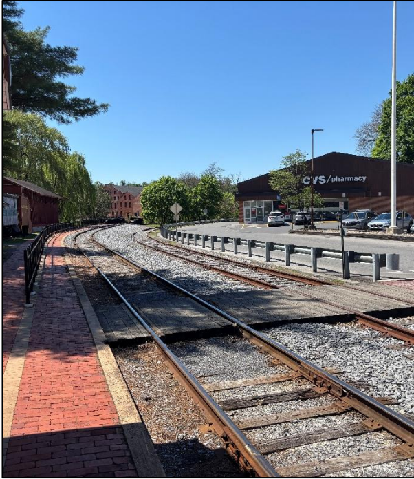
Photo 1 – Corridor from Talleyrand Park terminus, Looking South
