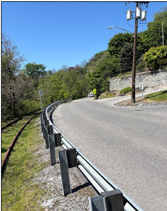
Photo 3 – South Potter Street shoulder, Looking West
