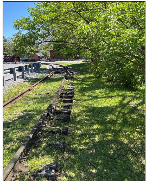
Photo 4 – Corridor near CVS Looking North
