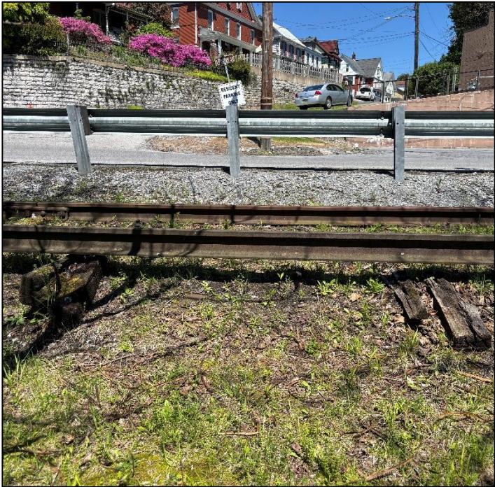
Photo 5 – Rail, shoulder, and South Potter Street, Looking North
